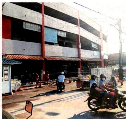
For many months, this gate facing Jalan Othman 4/40 served as the only entry/exit to the market, forcing customers to take a longer route and delivery trucks to wait longer.
